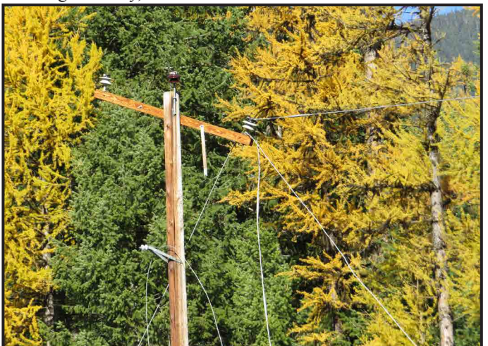
Left: A pole in the distance broken by a tree. Right: Broken wire and crossarm damage caused by a tree.
